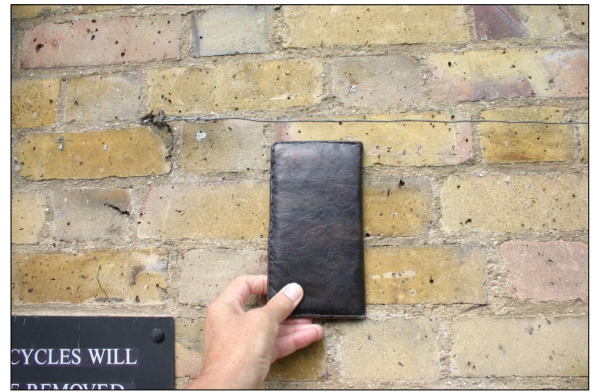
Fig. 6. Using a convenient object as a makeshift size reference: in this case, a wallet.
