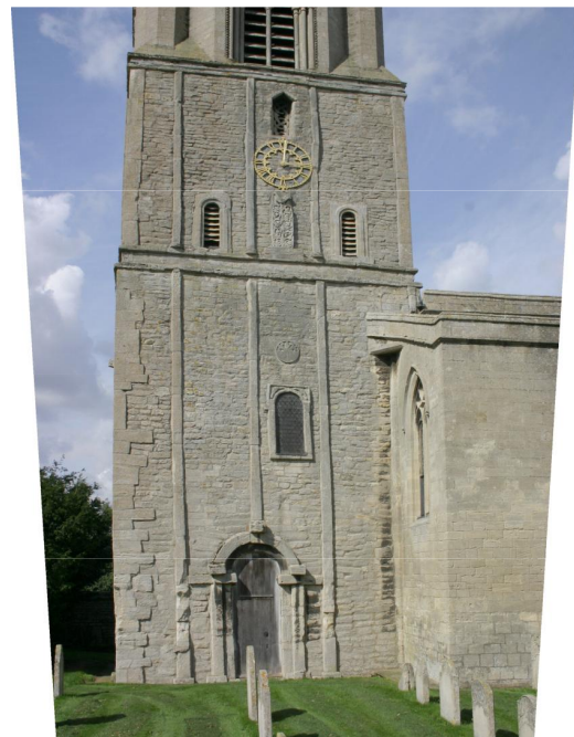
Fig. 2. Picture of the Anglo-Saxon dial (just above the lower window) at Barnack, Cambridgeshire. The image has been distorted so that vertical lines are now parallel. The dial width can easily be related to a measurement of the door at ground level. There is also some spherical distortion caused by the camera lens but this has been ignored here.
